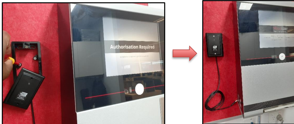
Mounting the RFID card Reader
